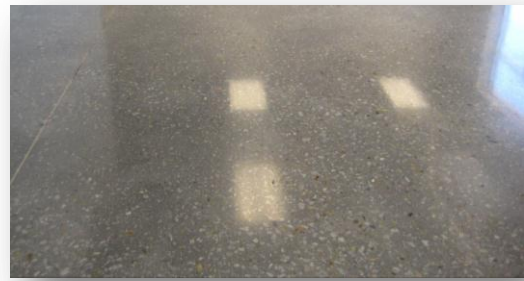
Illustration: Concrete floor
