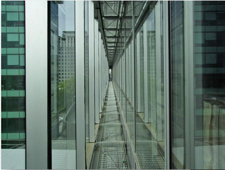
Illustration: Double skin façade and its cavity
